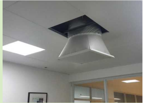
Connection between DiffuSox™ & inflow duct
