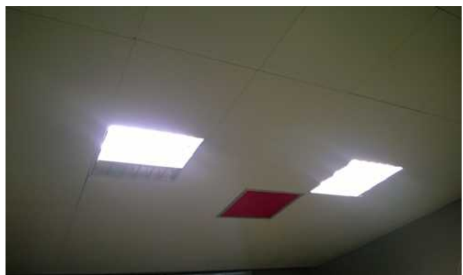
Offices with false ceiling
